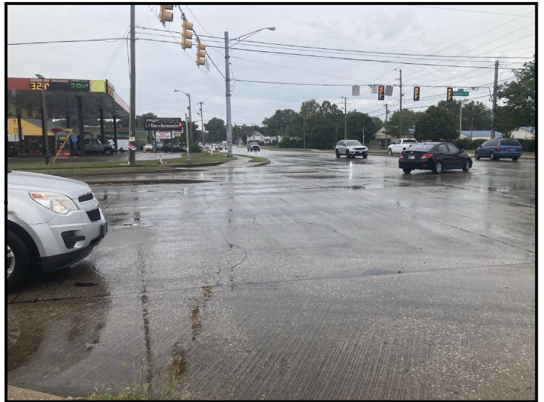
04 - Looking northwest from the southeast quadrant
