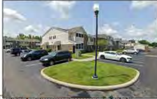
Echo Ridge Apartments
