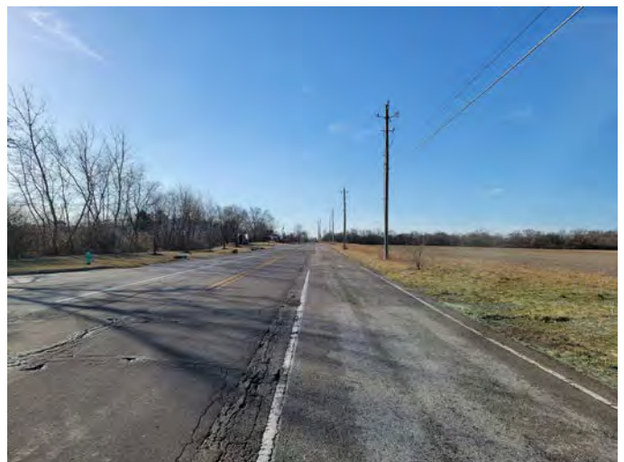
Franklin Road looking South towards Southeastern Avenue
