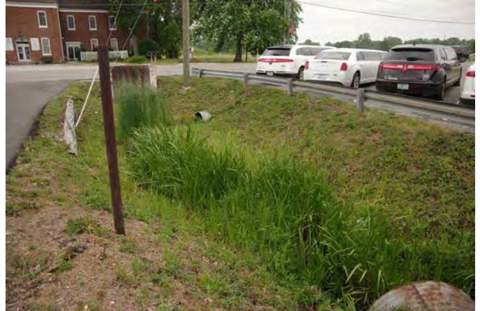
Stormwater Swale alongside Southeastern Avenue
