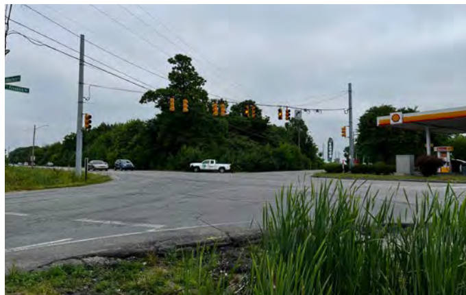
EXISTING - Intersection of Franklin and Southeastern Avenues which is not pedestrian or bike friendly
