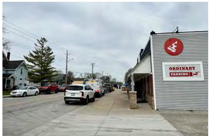
Existing sidewalk along Southeastern Avenue
