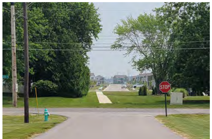
New subdivision south of Thompson Road with a dead end sidewalk
