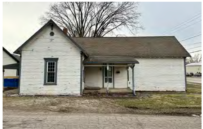
1880 Gothic Revival (Under Restoration)
