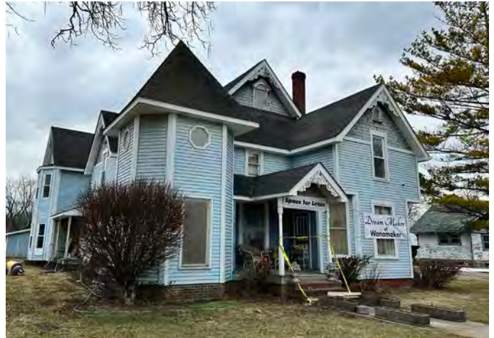
1890 Victorian with an addition in 2000
