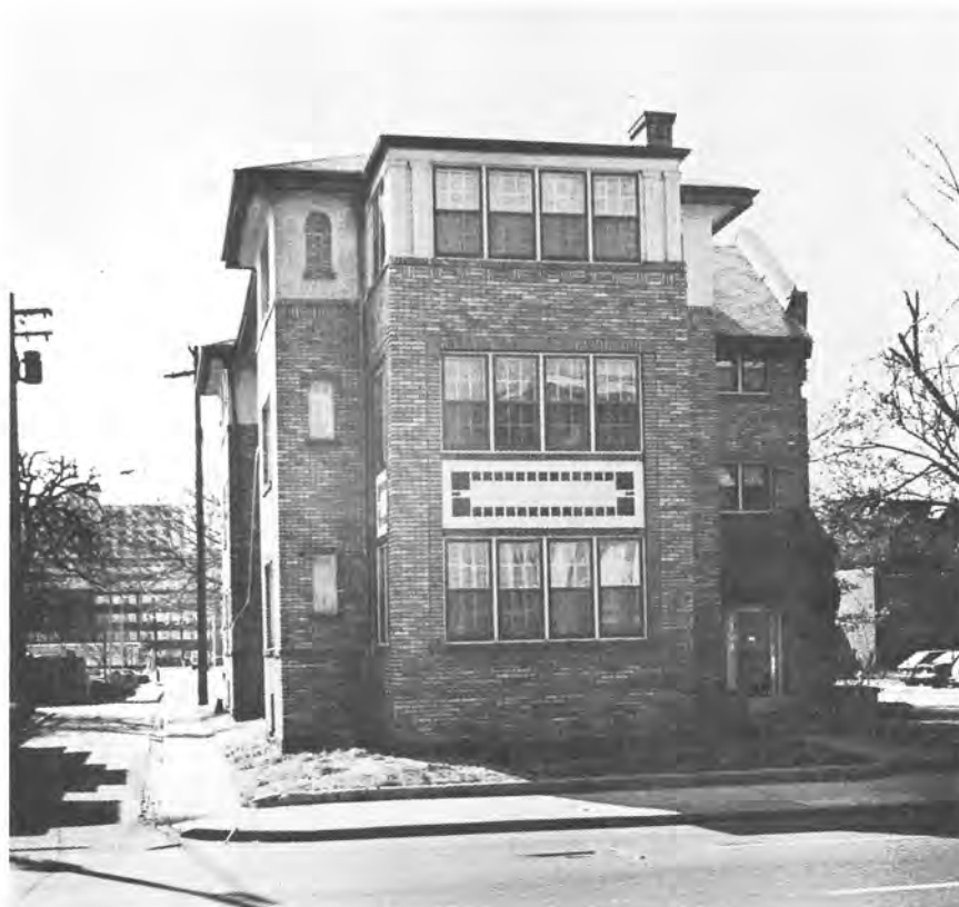
The Allen Apartments 1704 North Pennsylvania Street 1913
