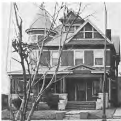
Wyon-Ashby House 1922-24 North Delaware Street 1897
