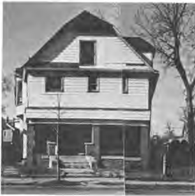
Vannice-Kriel House 1642-1644 North Alabama Street 1882
