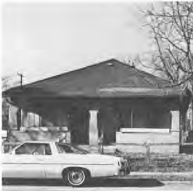
Noble-Conner-Banta Double Residence 1626-1628 North Alabama Street c. 1880
