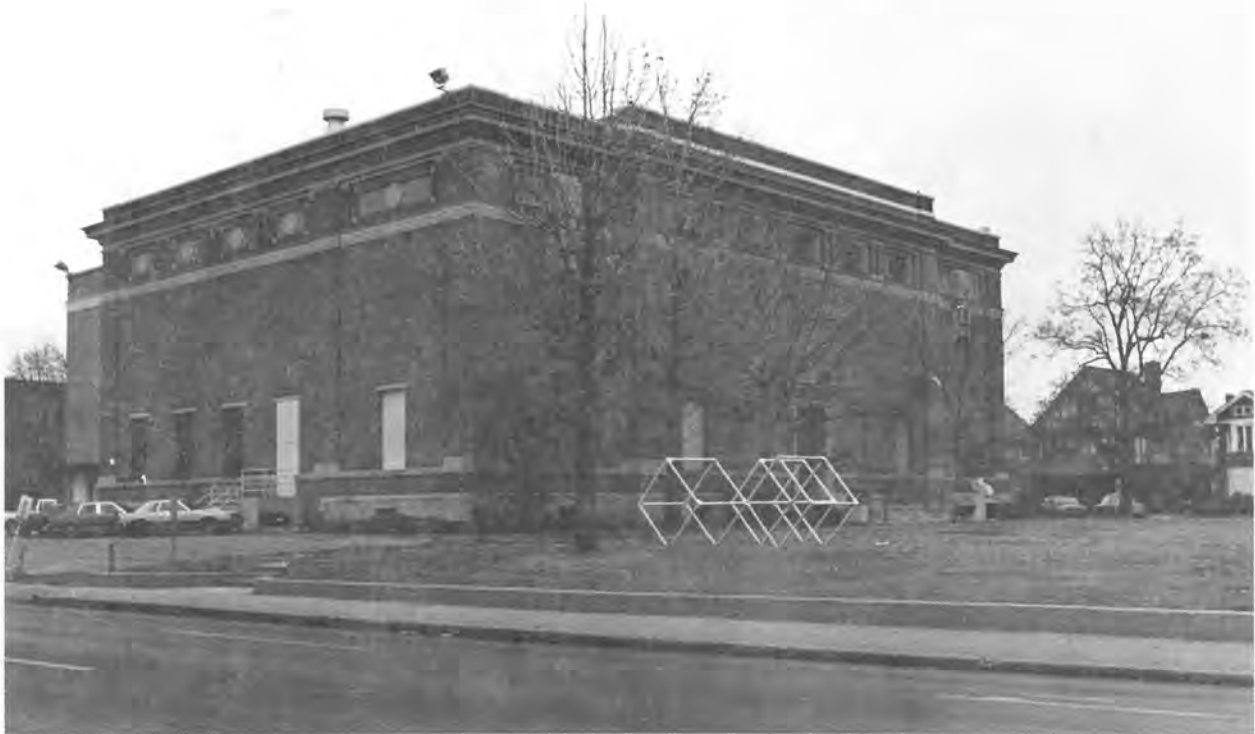
Herron School of Art 1701 North Pennsylvania Street 1906, Vonnegut and Bohn, architects
