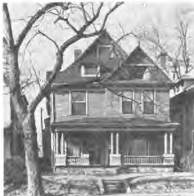
Smith-Keating-Carroll House 1930 North New Jersey Street 1897
