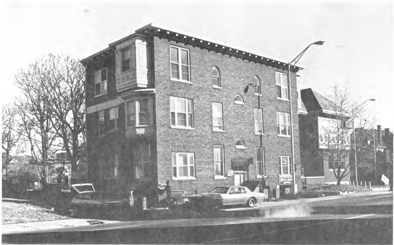
East Sixteenth Street Apartments 150 East 16th Street c. 1890 and c. 1920
