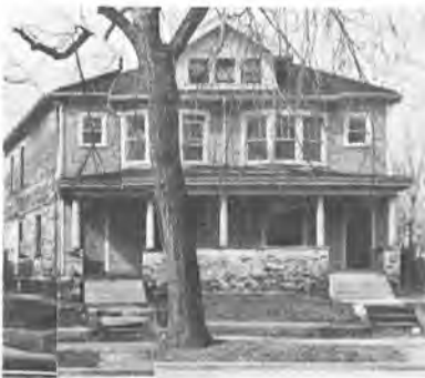
Carson-Tuck Double Residence 1838-1840 North Talbott Street c. 1910
