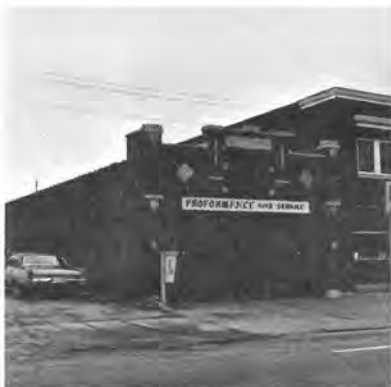
Peter Pan Building 1828 North Central Avenue c. 1923
