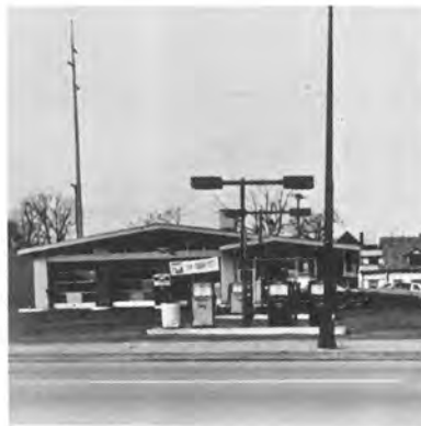
Service, Gas Station 2158 North Central Avenue c. 1965
