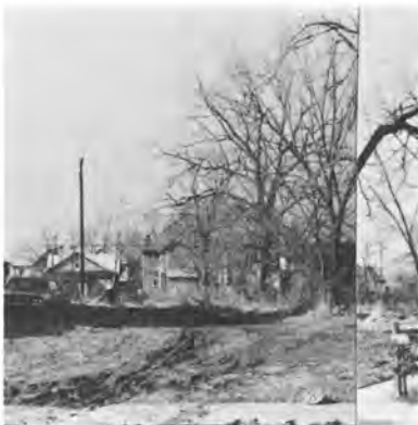
Vacant Lot 1818 North New Jersey Street
