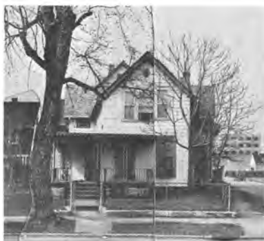
Lloyd-Sullivan House 1730 North Talbott Street c. 1885
