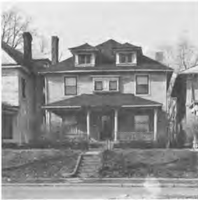
Hice-Kelly House 2126 North New Jersey Street c. 1907
