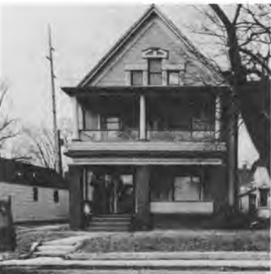
Rehm-Runyon-Willis Double Residence 2060-62 North Central Avenue c. 1897
