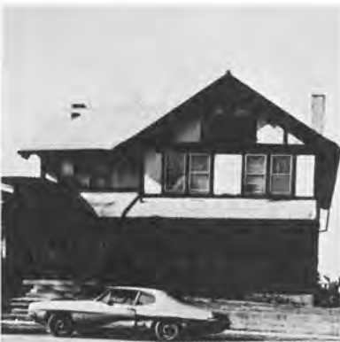
James Burks Double Residence 2064-66 North Alabama Street c. 1914
