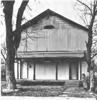
Pye Double Residence 1622-1624 North New Jersey Street c. 1882
