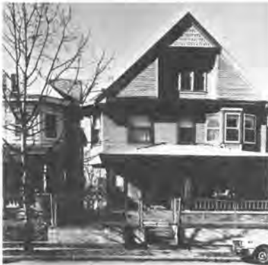
Hess-Hetherington House 2052 North Alabama Street 1898
