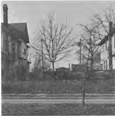
Vacant Lot 2108 North New Jersey Street
