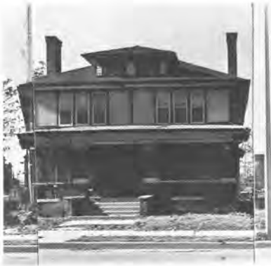
Gocke Double Residence 2156-2158 North Pennsylvania Street c. 1909
