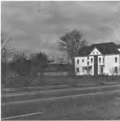
Vacant Lots 1912 to 1926 North Alabama Street
