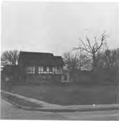
Vacant Lots 2140 to 2158 North Alabama Street
