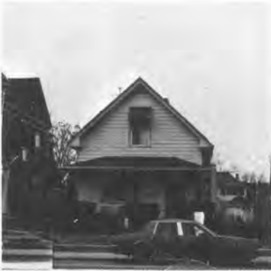
Harper-Church House 1644 North Delaware Street 1880
