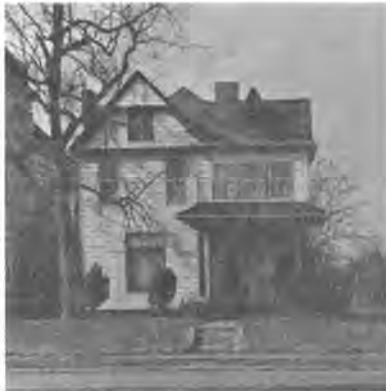
Webb-Maxwell House 2020-22 North New Jersey Street 1894
