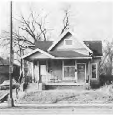
Brady House 2012 North Central Avenue 1895
