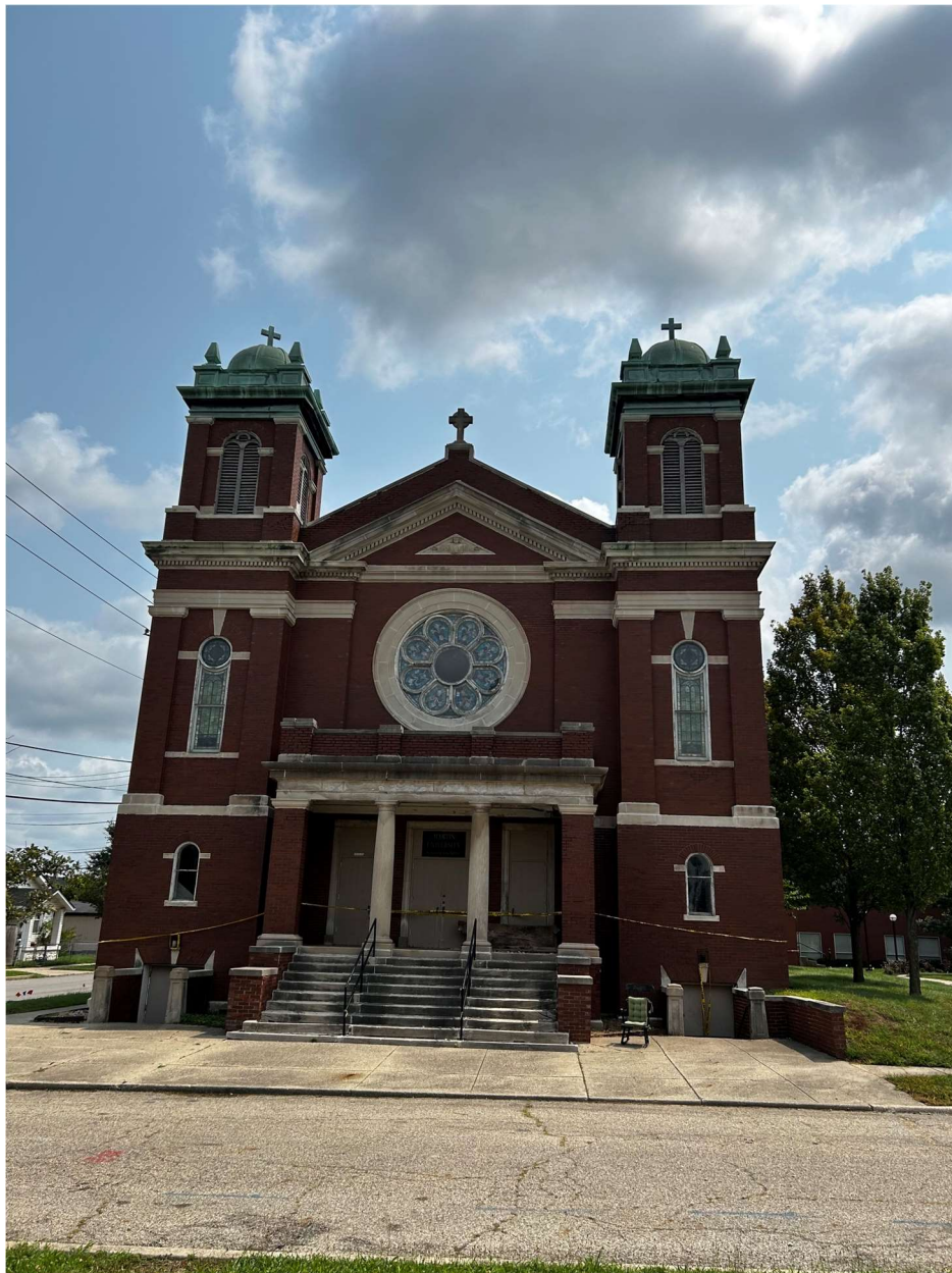
Front (west) facade
