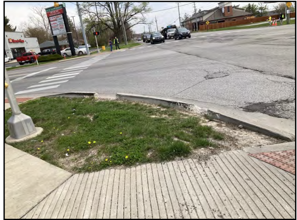
Looking east from NW quadrant
