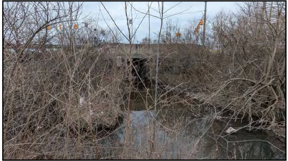
North side of bridge looking south
