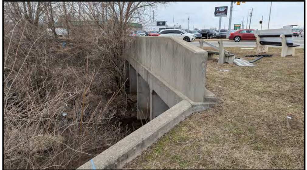
Bridge headwall in southeast quadrant
