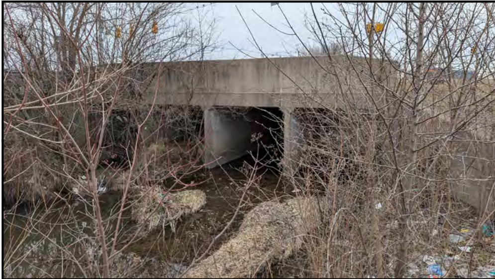
South side of bridge looking north
