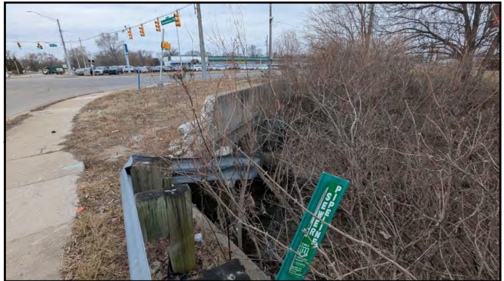
Looking north from bridge in northwest quadrant
