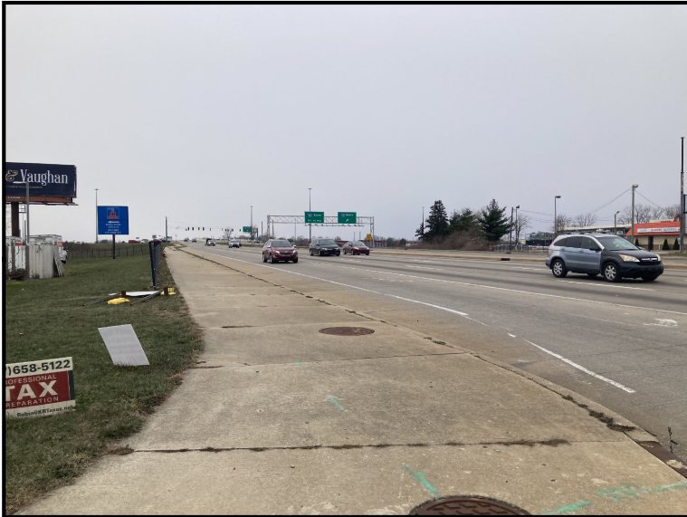
Looking west on 38th St. from the SW corner
