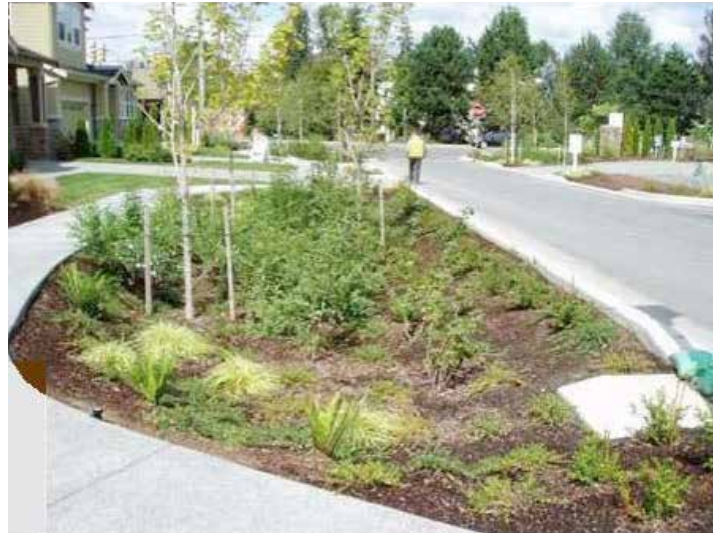
A residential rain garden
