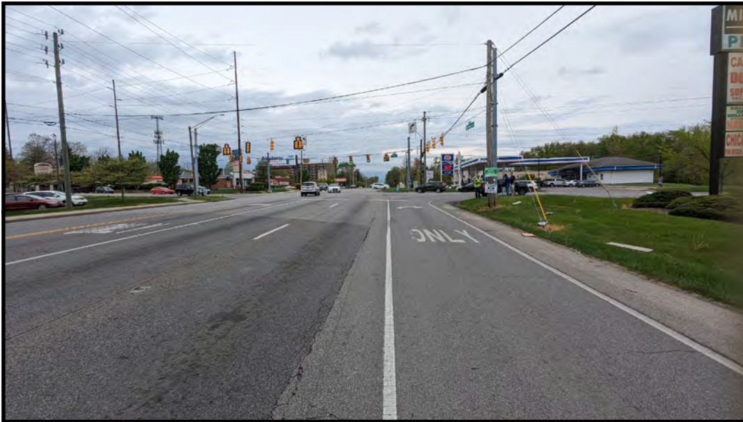
Arrow pointing at the raised curb showing the shift in alignment of Michigan Road looking northbound.
