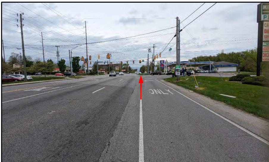
Photo 2 – Arrow pointing at the raised curb showing the shift in alignment of Michigan Road looking northbound.
