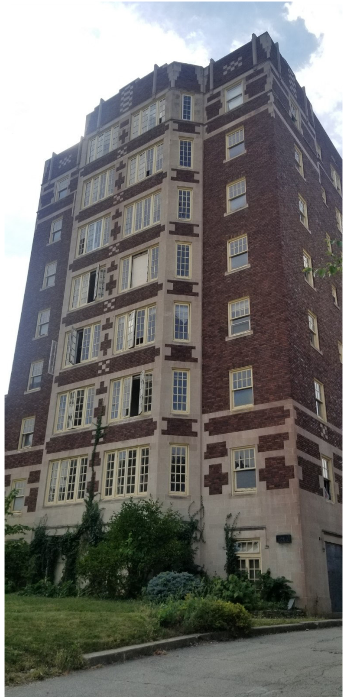
Fig.4 East and partial north elevation. Photo: IHPC Staff, 2019
