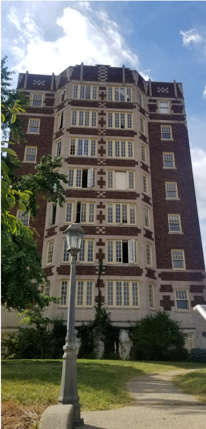
Fig.1 East elevation. Photo: IHPC Staff, 2019
